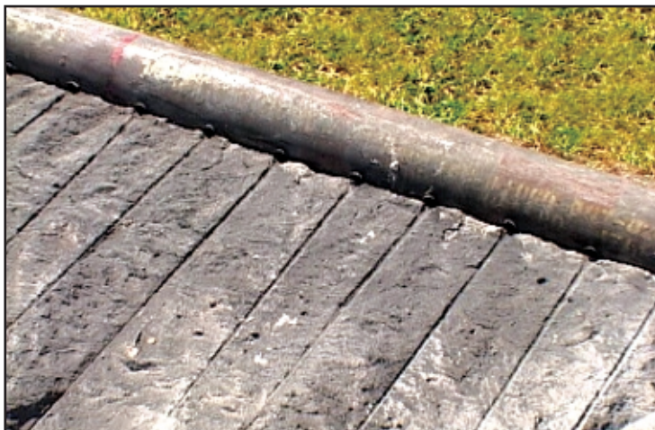
Perforation testing ensures optimal performance.
